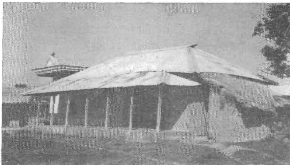
A MUD-WALLED HOUSE WITH ROOF OF C. I. SHEETS
